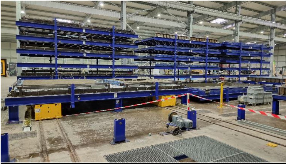
Image 6: A lifting beam takes over the circulating pallet for the curing process and stacks them in the desired intermediate storage position on.
