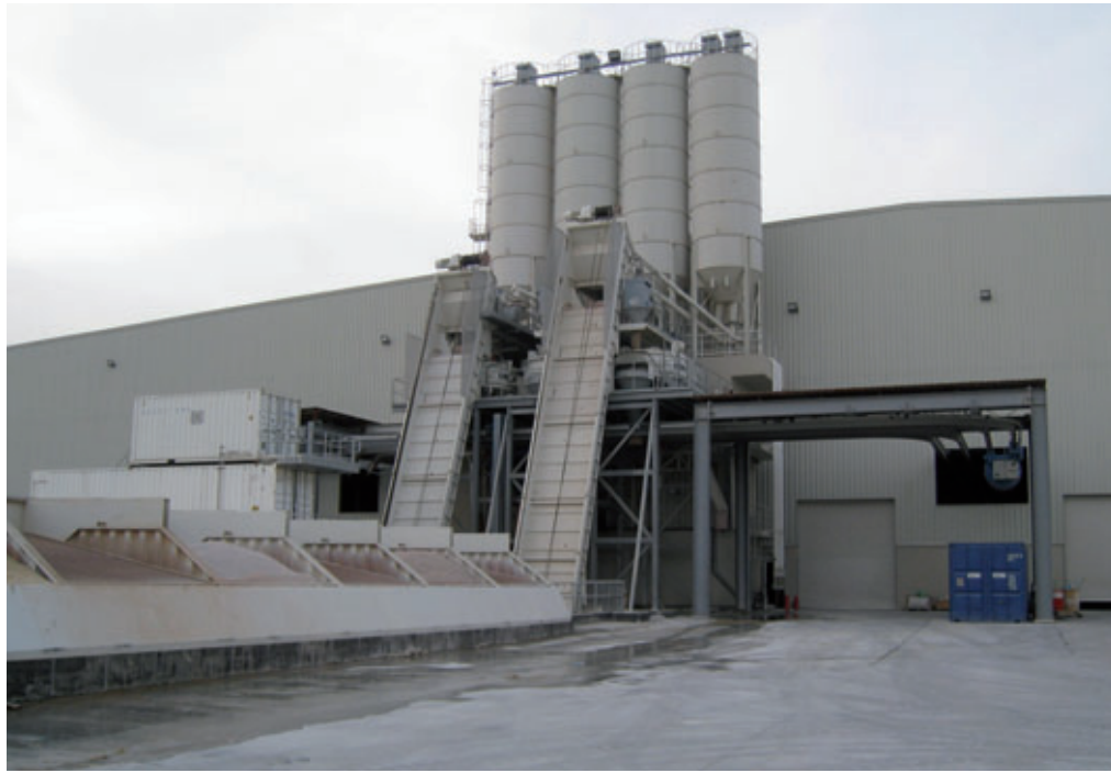
Batching Plant and Concrete Delivery System
