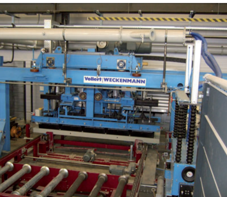
After the specified hardening period, the blocks are automatically removed from storage by a storage and retrieval system and conducted to the stripping manipulator
