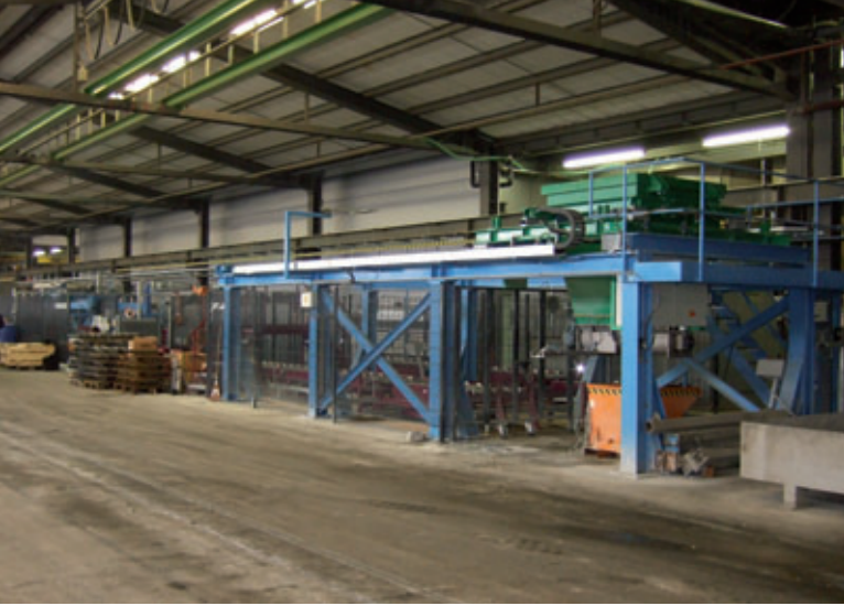
Concreting takes place with self-compacting concrete using a spreader at the concreting station
