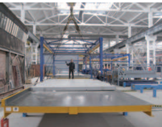
Lifting the finished flooring slabs with a gantry and subsequent transport to outside storage on a platform carriage
