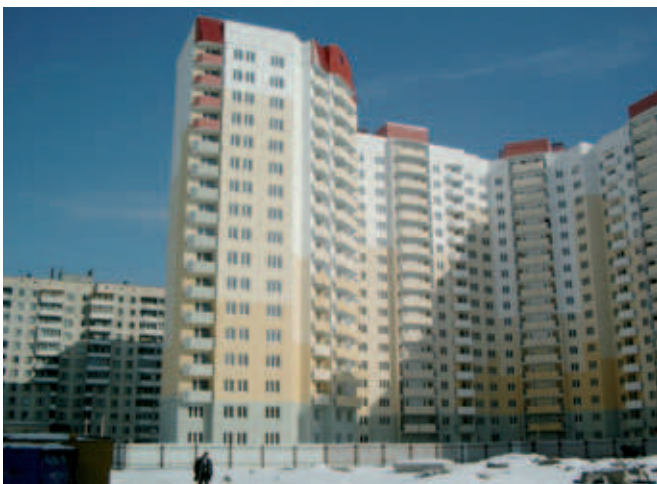
The construction method with massive walls and heat insulation cladding possesses considerable advantages as construction progress can be accelerated and no joint appears on the façade
