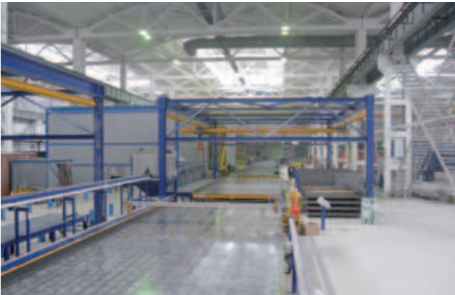
The pallet circulation system is equipped with 40 pallets (3.9 x 12.5 m) which have edging formwork fastened with screws on the longer side
