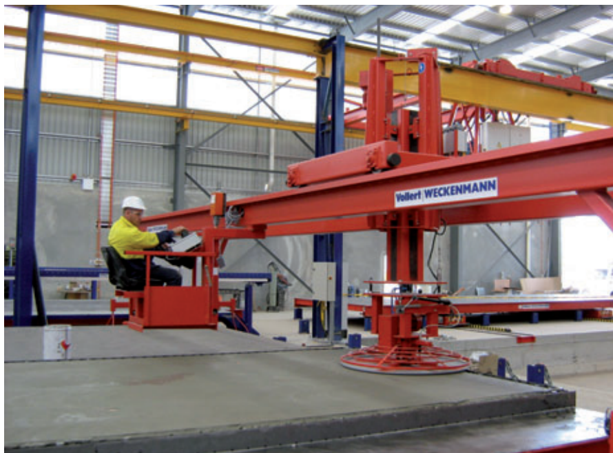
Fig. 18: Floating the concrete surfaces
