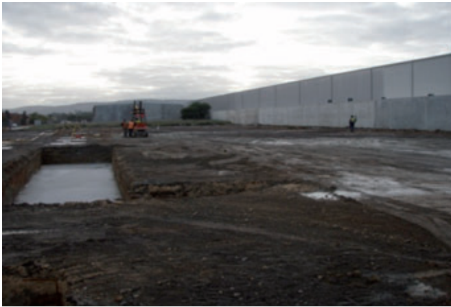
Fig. 4: Preparation for the foundation works
