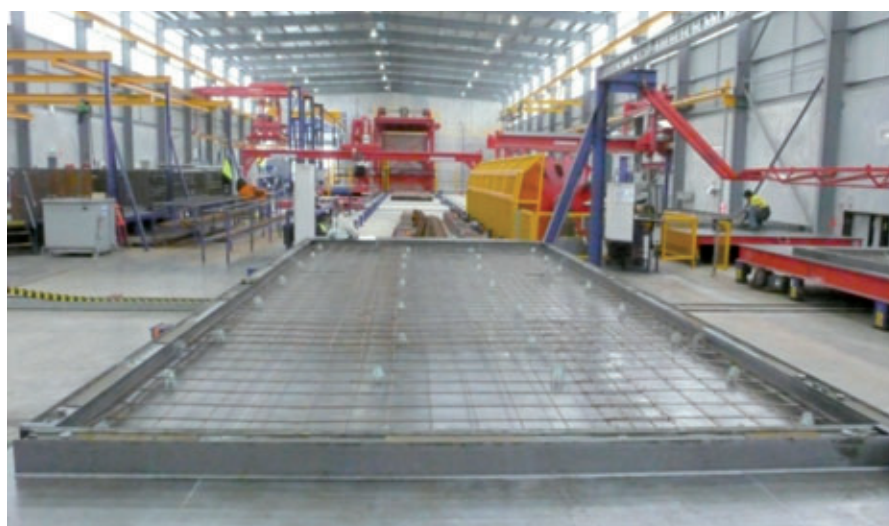
Fig. 15: Insertion of the reinforcement
