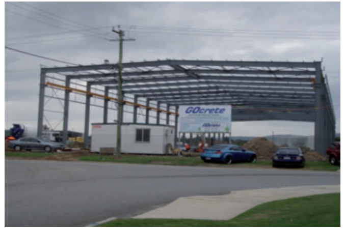
Fig. 5: Steel structure of the hall
