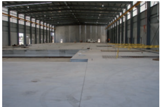
Fig. 7: Completion of the floor plate
