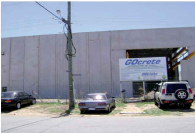
Fig. 6: Hall cladding with precast concrete components
