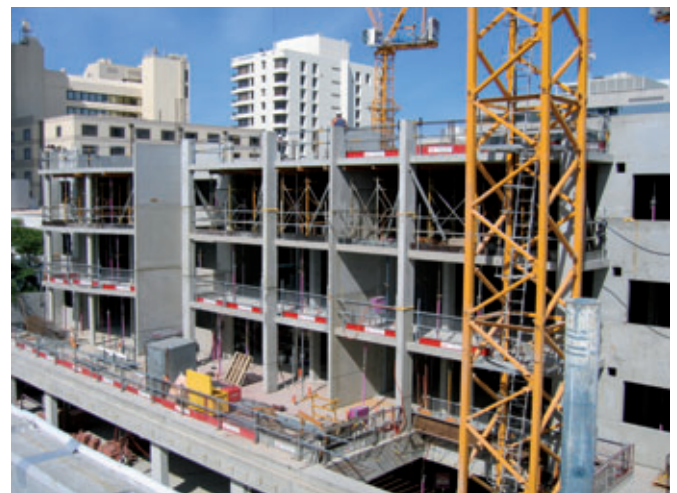
Fig. 3: Apartment house in Perth under construction
