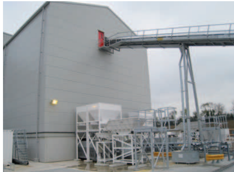
Fig. 36: Skako Concrete Batching Plant
