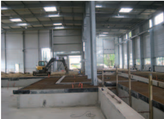
Situation during the manufacture of the foundation slab
