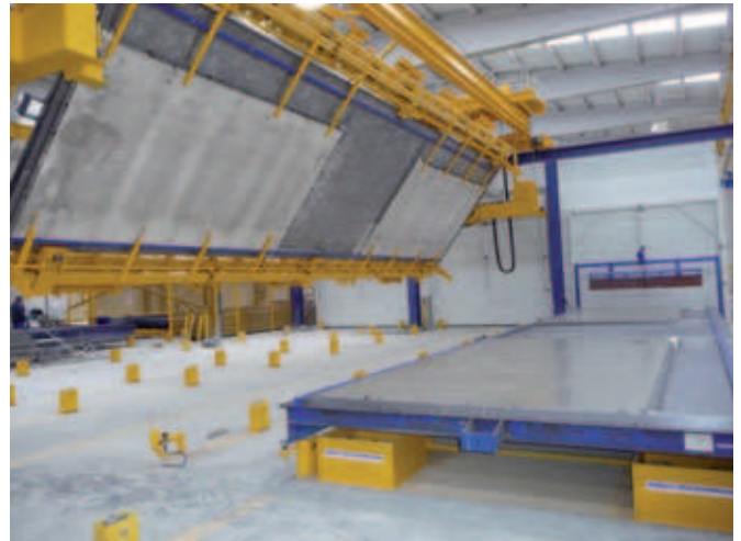
Turning machine during turning in / situation after the extension
