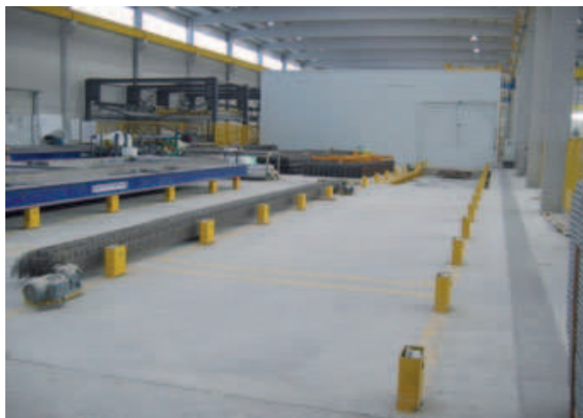
Situation before the installation of the turning unit and vibrating station
