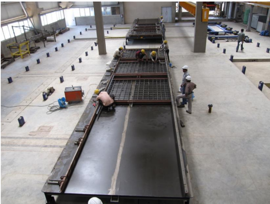
Fig. 6: Fitting the reinforcement
