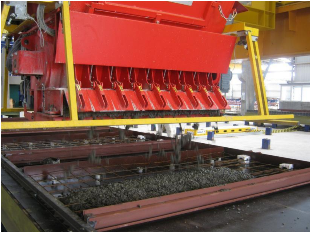
Fig. 8: Discharging fresh concrete on to the pallet
