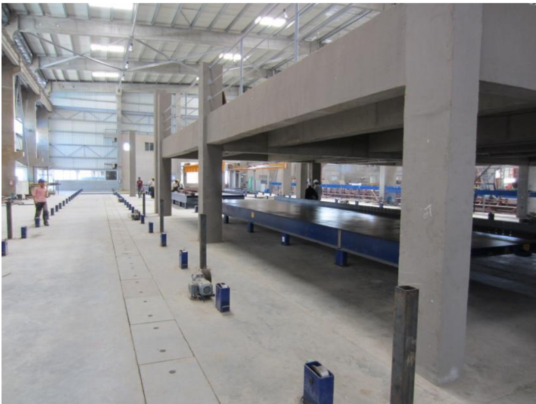
Fig. 10: Parallel production lines permit flexible precast concrete part production
