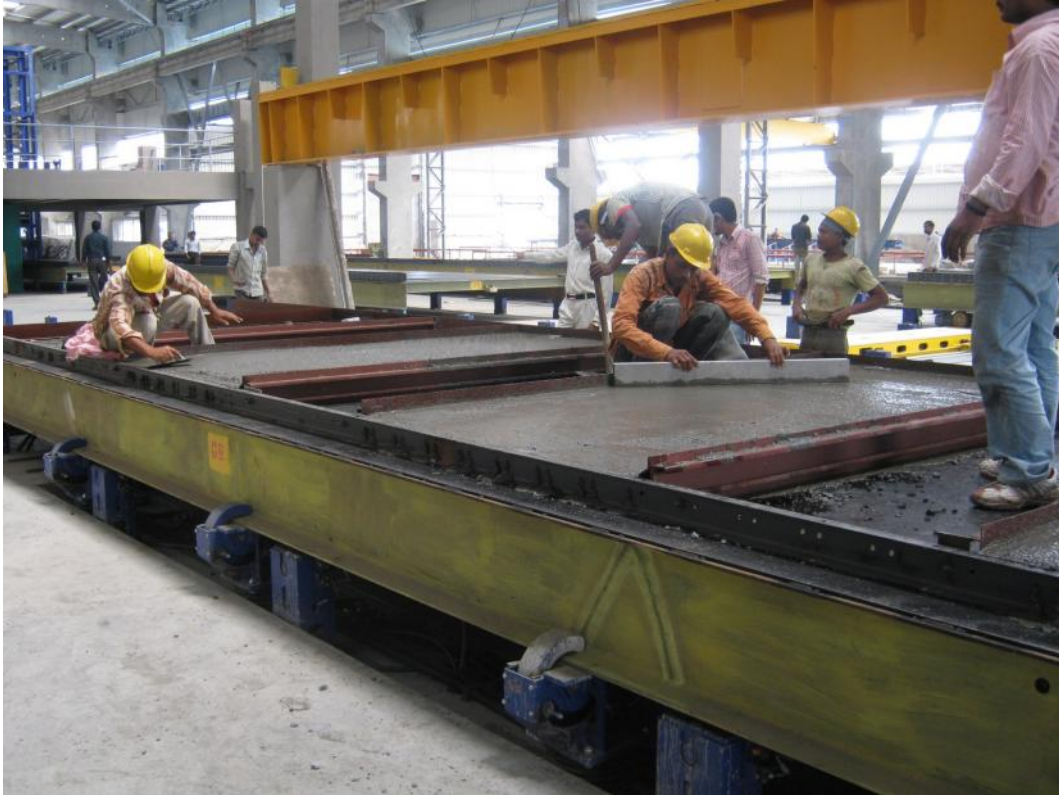
Fig. 15: Manual trowelling of the concrete surface
