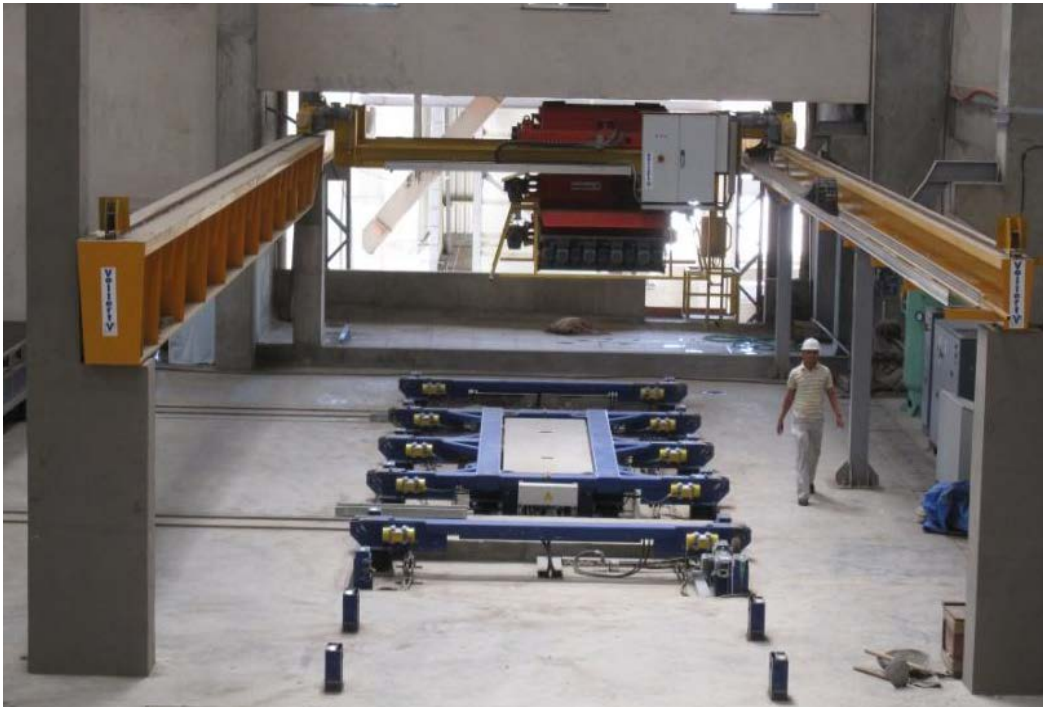
Fig. 9: Combined vibrator/shaker station for compacting the concrete
