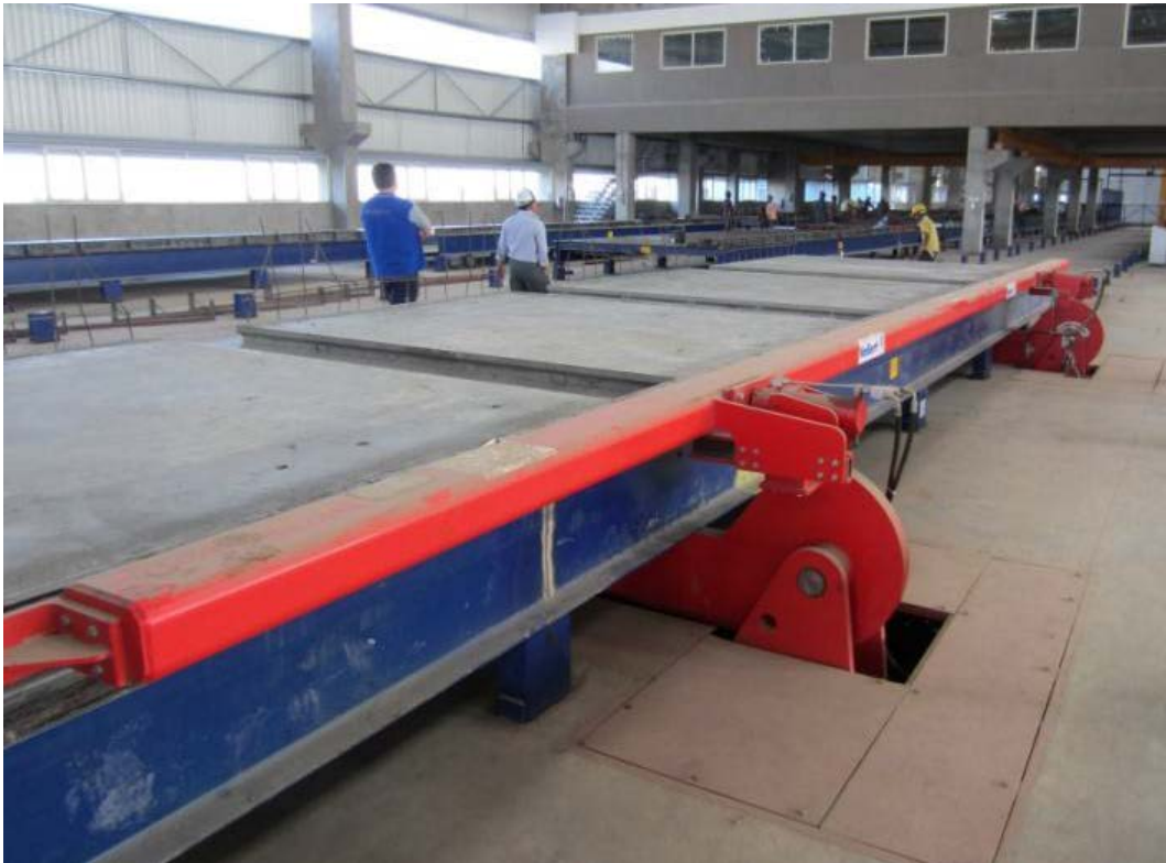
Fig. 16: Tilting table for stripping of the solid walls and solid slabs
