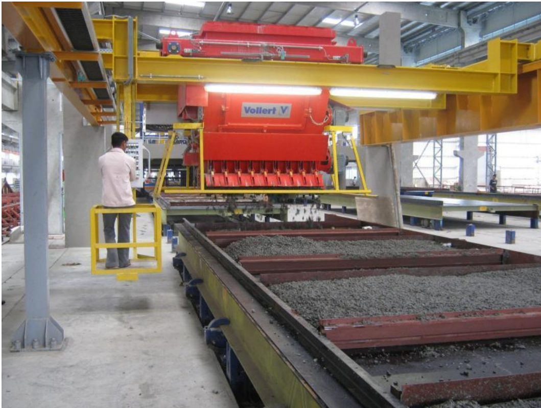
Fig. 7: Concrete spreader with mobile operating platform
