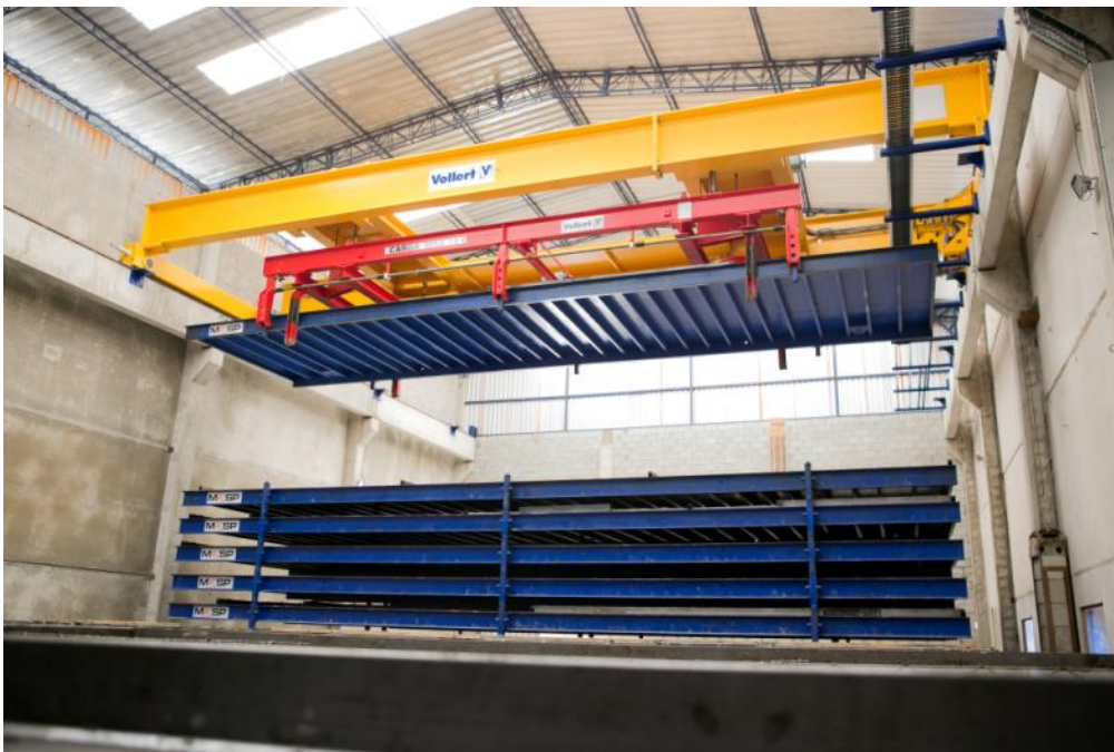
Fig. 4: Through the modern curing process alone it was possible to considerably shorten the turn-around times between concreting and demoulding
