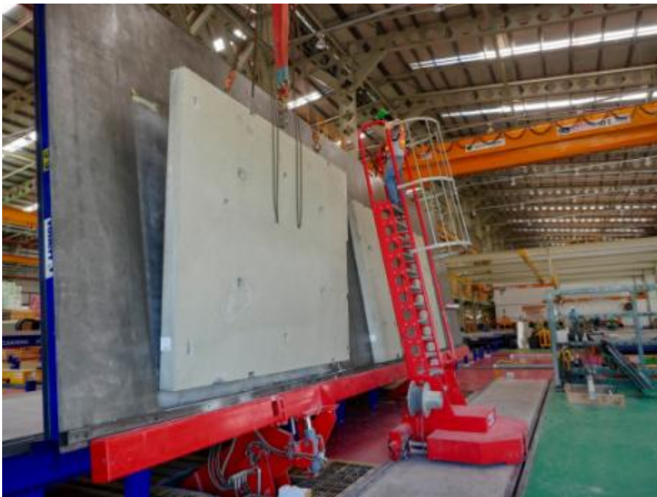
Fig. 10: The vertical lifting of the solid concrete elements is performed by two high-performance tilting stations
