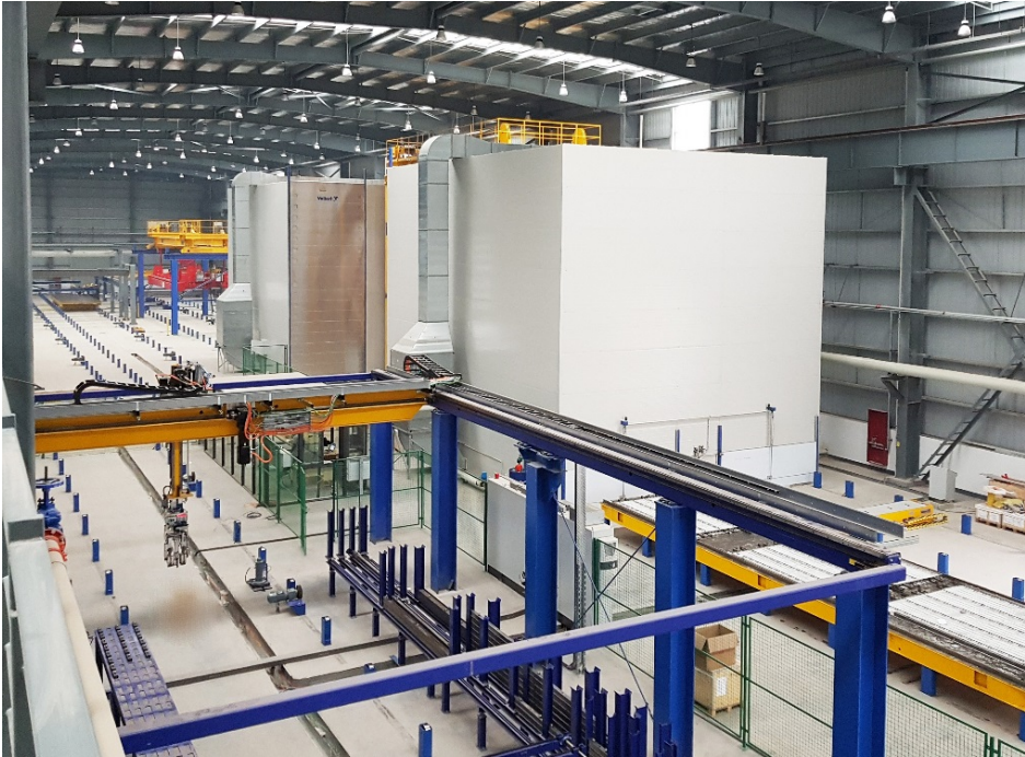
Image 1 The new precast concrete production line in Quzhou will increase the capacities of the Baoye Group by 700,000 m 2 of wall and slab elements per year.
