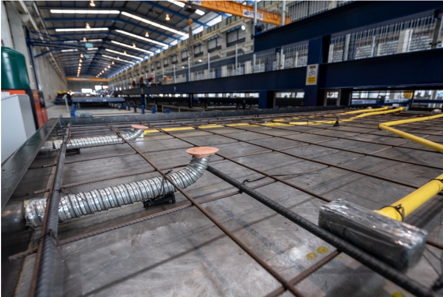
Image 4 (Source: DSC Product) The total of 30 pallet positions are integrated via a VARIO SHIFT central shifter platform as the core element.
