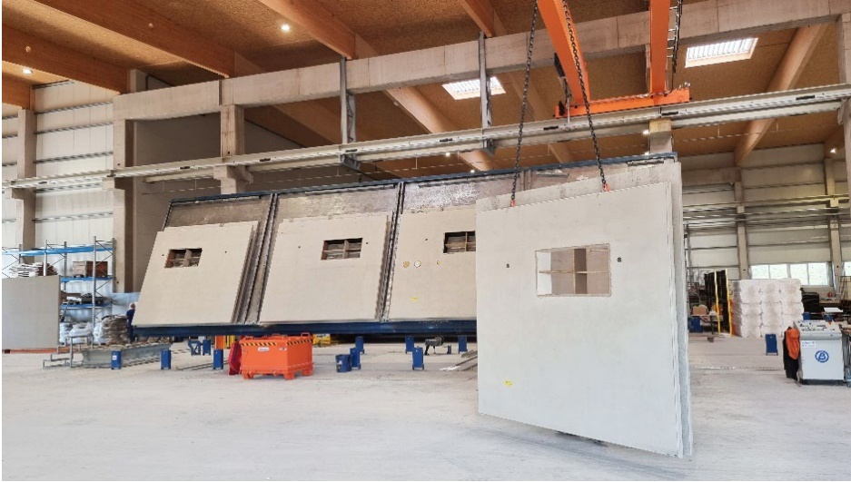
Image 9: A Vario TILT tilting station lifts double walls vertically.
