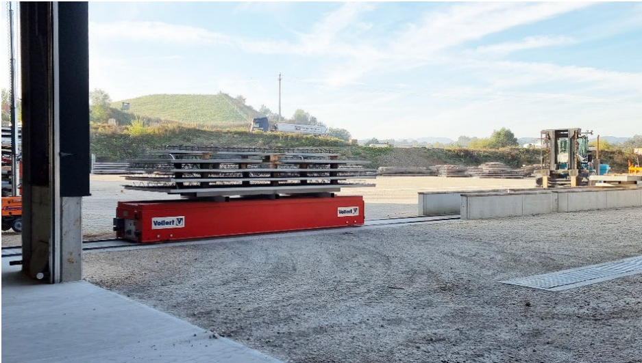
Image 10: The slab stacks are transported outside by a removal truck.
