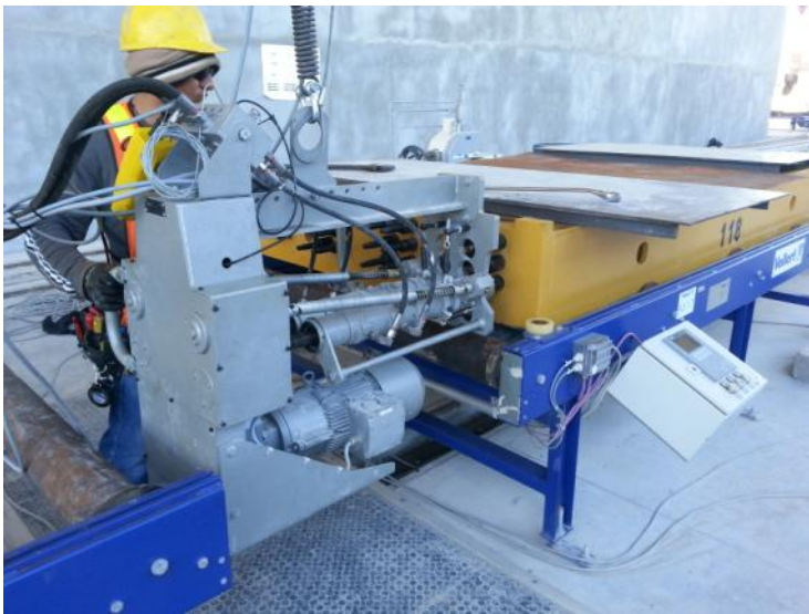
Fig. 2: Subsequently, the wires are prestressed by means of the tensioning bolts whilst constantly monitoring and recording the tightening torque of each prestressing wire.
