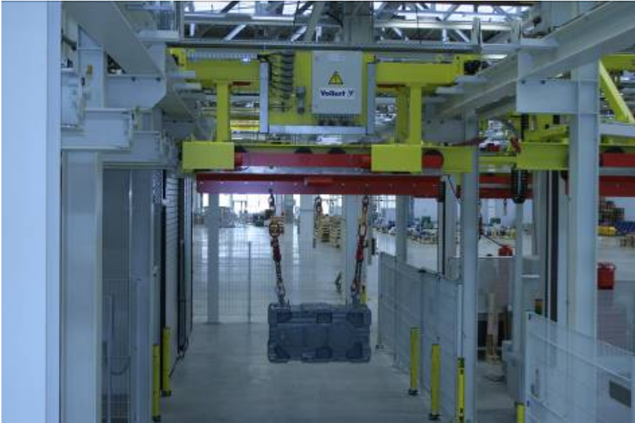
Image 5 After drying, the finished large gear units are lowered by two lifters with integrated weighing equipment on pallets or on transport crates and taken directly to the logistics department.
