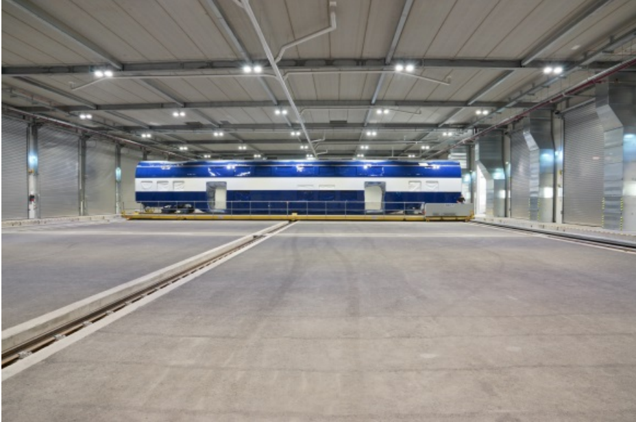
Image 1 In the new Siemens AG Austria coating center, metros and passenger carriages are automatically transported from a central transport system to the individual coating treatment booths.
