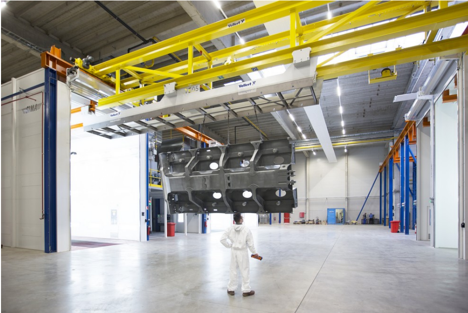
Image 1 Faymonville has opted for a double-track over-head conveyor with wheel and disk drives for coating. The workstations arranged in parallel ensure a space-saving plant layout.
